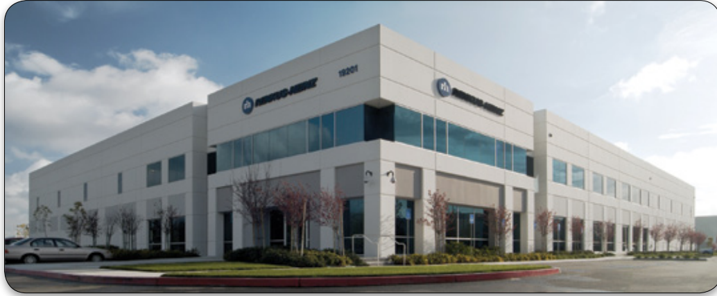
Renkus-Heinz, Inc. Headquarters, Foothill Ranch, California, USA
